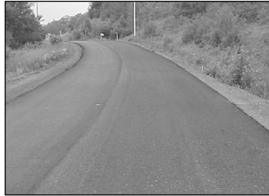
1b. Finished Mat – RAP Cold Mix
