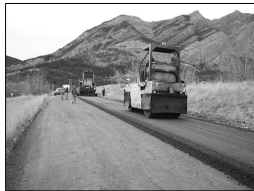
2b. Placement and Compaction
