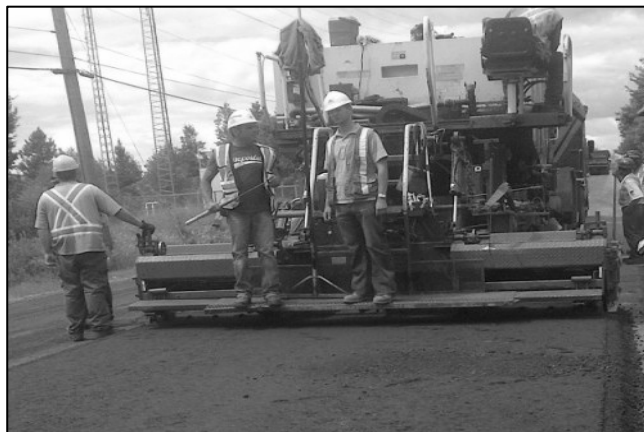
Figure 4: Lay Down of 100% Reclaimed Asphalt Pavement (RAP) Cold Mix
