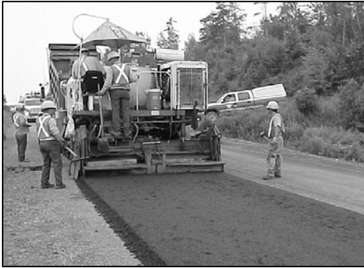
1a. RAP Mix Placement
