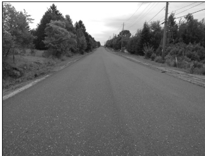
Figure 6. Finished Pavement Surface After One Month
