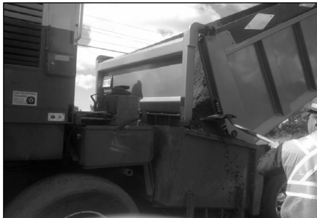
Figure 3. Midland Paver with 100% Reclaimed Asphalt Pavement (RAP) Mix
