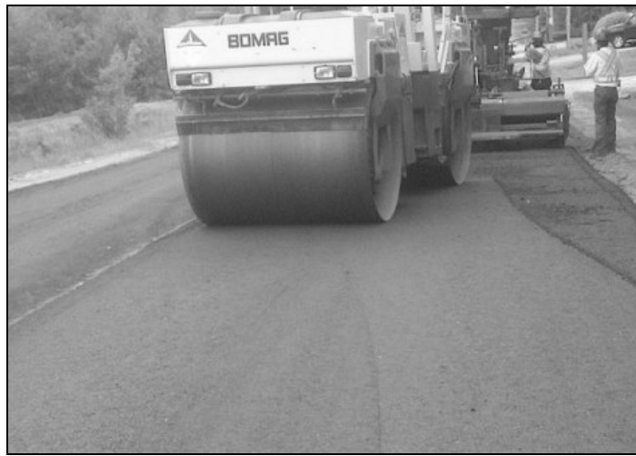
Figure 5. Compaction with Double Steel Drum Roller
